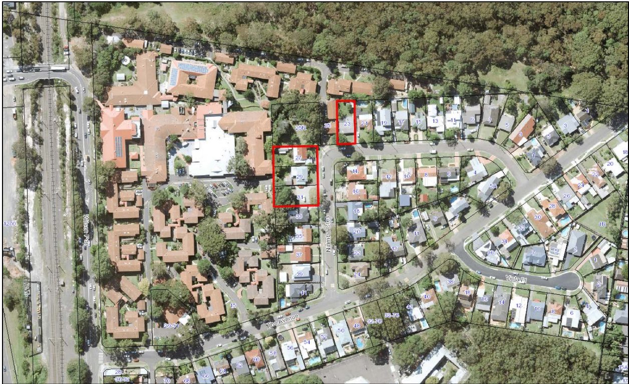
Figure 5: Nirimba Crescent, Heathcote (subject properties outlined in red)
